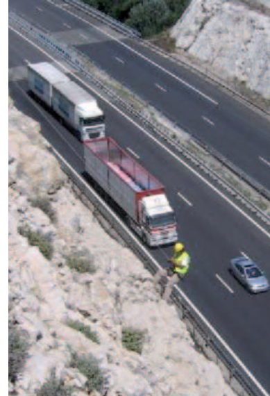
Diagnostic falaise - Autoroute A9
